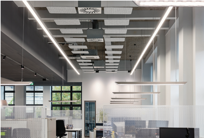
Acoustic pads from the Rossoacoustic PAD product family were installed under the ceiling to absorb sound. Photo: Jörg Hempel
