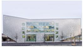
The Futurium is an energy plus building in terms of its primary energy consumption, thanks to its compact design, passive construction measures appropriate for the usage of the building (the building envelope in particular) and a strict policy of needs-based air and energy provision as well as highly-efficient building services technology. Photo: Dacian Groza, Berlin
