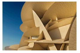
The building is composed of 539 different disc-shaped elements, each with a diameter of up to 87 metres. The discs are arranged in a staggered fashion, partially overlapping one another. Image: Andreas Keller, Altdorf
