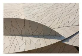
DA detail view of the staggered disc-shaped elements, evoking the crystalline structure of a desert rose. The realization of the challenging construction design required a superior level of technical expertise from the Werner Sobek engineering team. Image: HG Esch, Hennef
